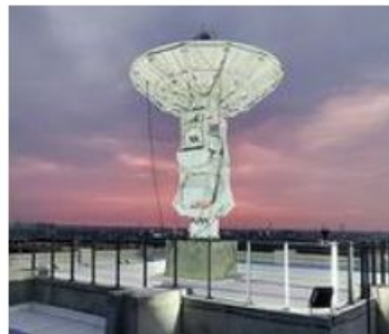
A view of Dhruva Space's 3.8m S&X-band ground station antenna in Hyderabad.
