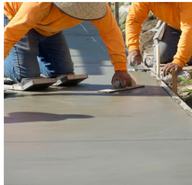
Construction workers putting finishing touches on freshly poured concrete. GETTY IMAGES
